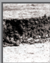
Roller compacted concrete
